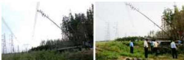
Fig.1. Green tree fall on the 500 kV line.
